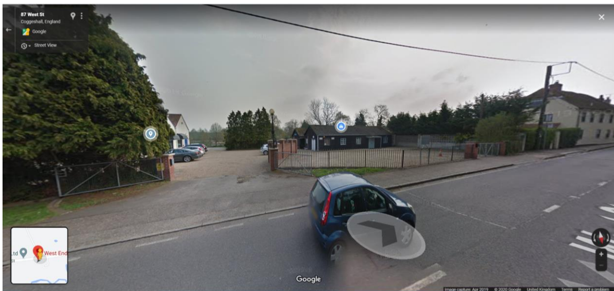
Google Street View from West Street of timber buildings on site
